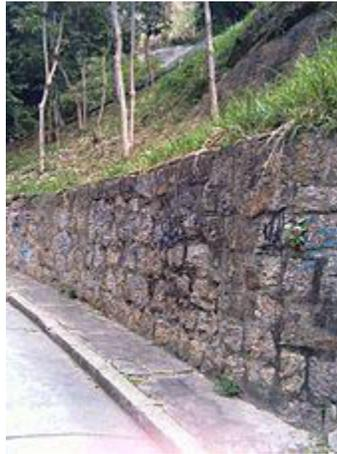
A retaining wall is a structure that holds back earth. Retaining walls stabilize soil and rock from down slope movement or erosion and provide support for vertical or near-vertical grade changes. Cofferdams and bulkheads, structures to hold back water, are sometimes also considered retaining walls.
